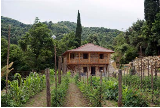
The Axion Estin Cell, a dependency of Pantokrator Monastery, is located not far from Karyes. Photograph of the completed phase 1, courtesy of Graham Speake, The Friends of Mount Athos
